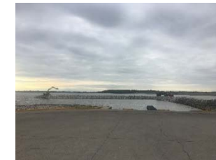
Flood Repairs Dam West Breakwater
