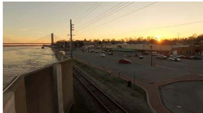
Cape Girardeau Floodwall
