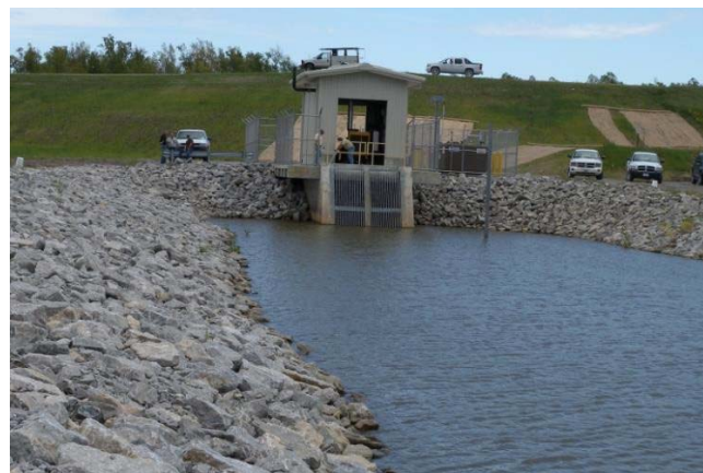
Missouri Chute Pump Station
