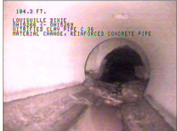
Photo: OH15269_OH15266124907_05112009_A.JPG, VCR No.: FLOOD WALL#2, 01:46:54 104.3FT, Material Change, Reinforced concrete pipe
