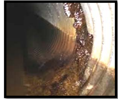
Deficiencies like corrosion (above left) and joint separation (above right) are commonly found in pipes operating past their life expectancy.
