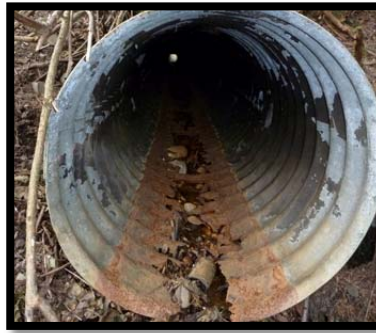
Deficiencies like corrosion (above left) and joint separation (above right) are commonly found in pipes operating past their life expectancy.
