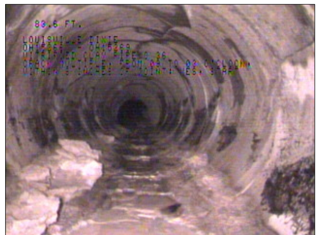
Photo: OH15269_OH15266124807_05112009_A.JPG, VCR No.: FLOOD WALL#2, 01:46:12 83.6FT, Crack Multiple, from 09 to 03 o'clock, within 8 inches of joint: YES, Start
