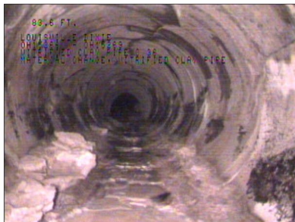
Photo: OH15269_OH15266124748_05112009_A.JPG, VCR No.: FLOOD WALL#2, 01:46:07 83.6FT, Material Change, Vitrified clay pipe
