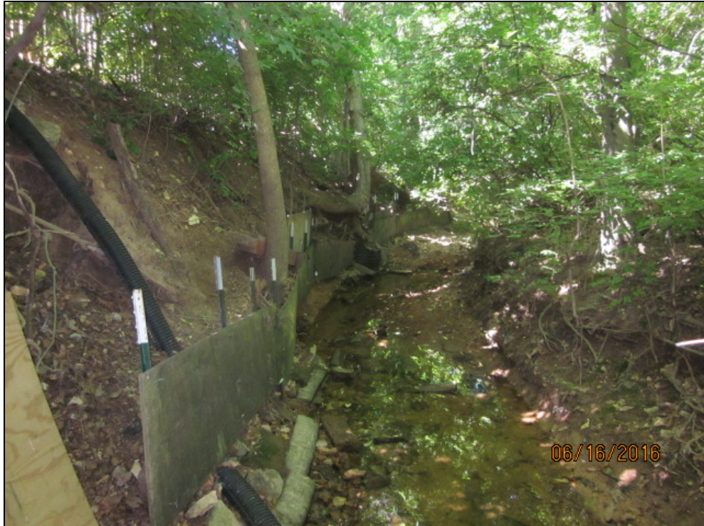
7- More plywood attempt at bank stabilization.
