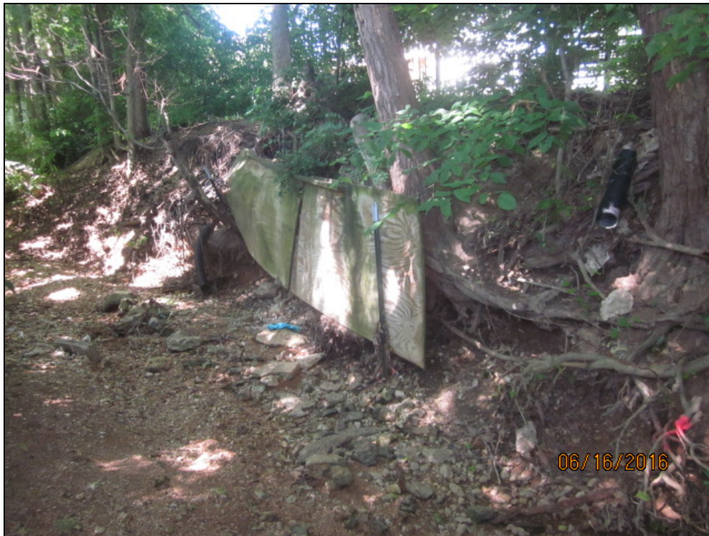
5- Stabilization attempted from plywood.
