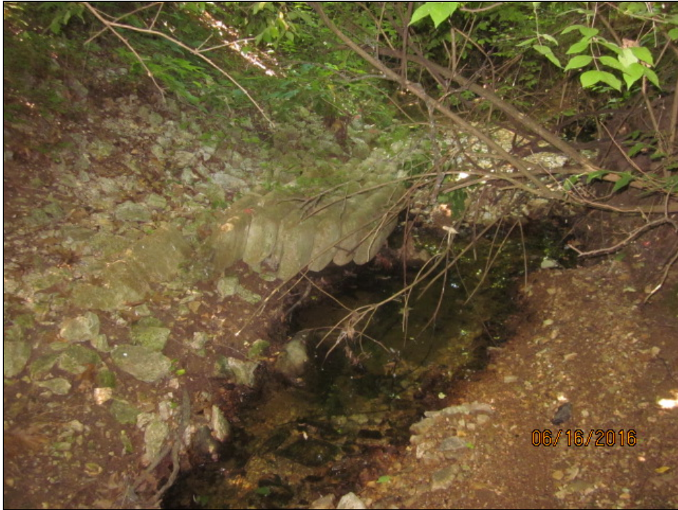
9- Failed concrete bag revetment.
