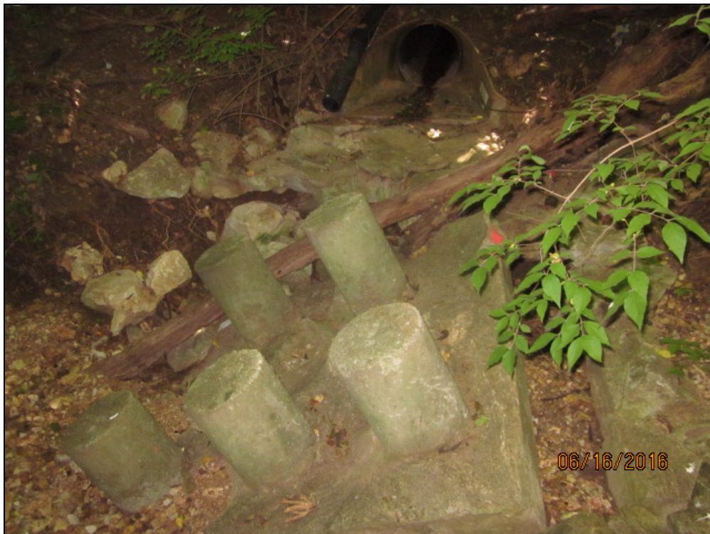
8- Separated energy dissipater at stormwater outfall.
