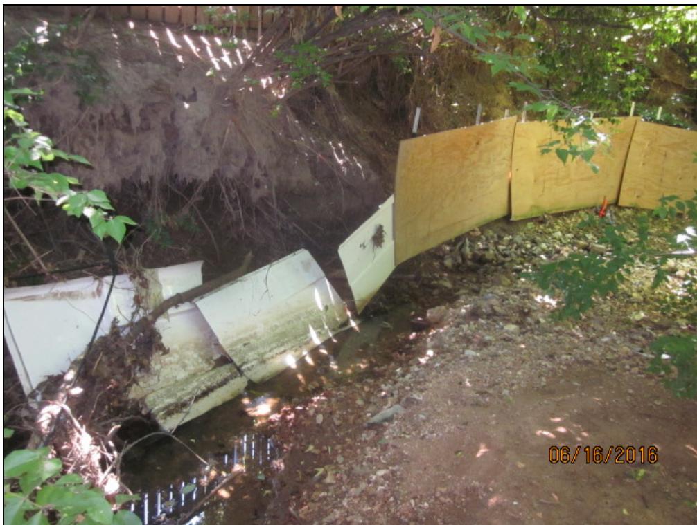
6- Stabilization attempted from plywood and sections of shower stall.
