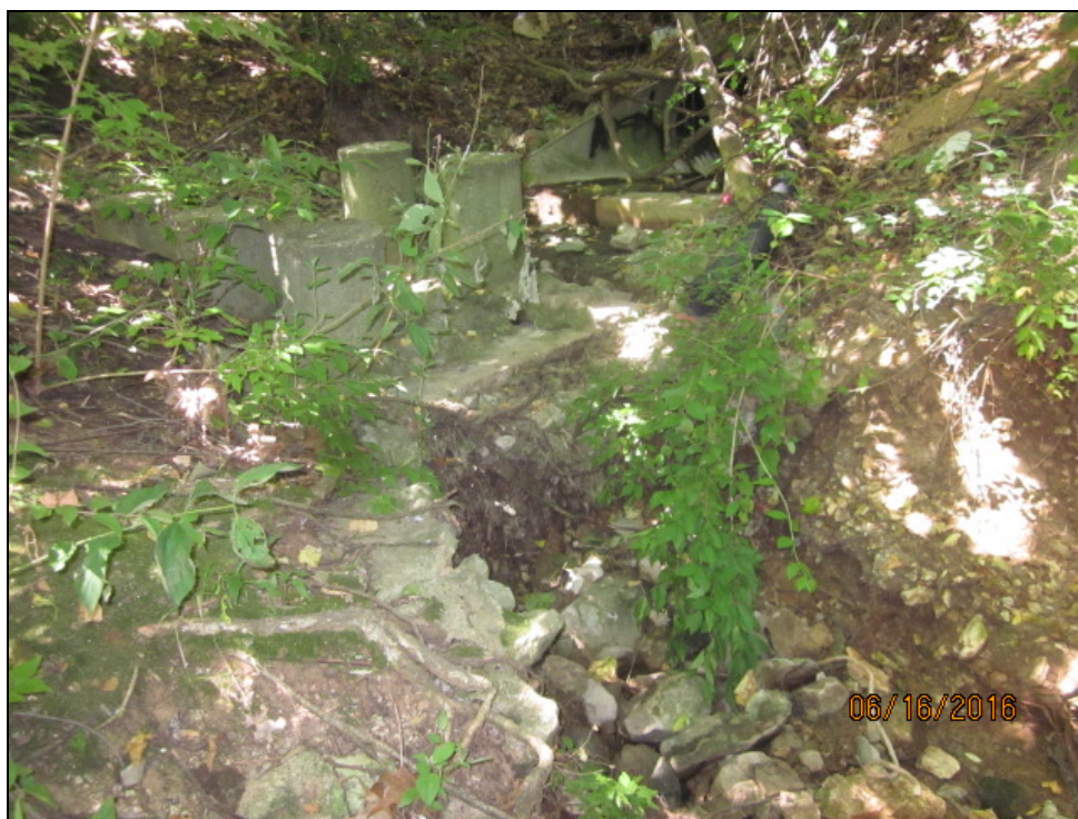
11- Failing stormwater outfall.
