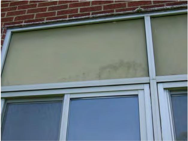
Moisture is Infiltrating in and around the Window Frames
