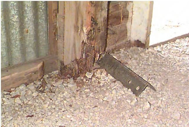
One of the main support beams in the Groves Building that is deteriorated at base
