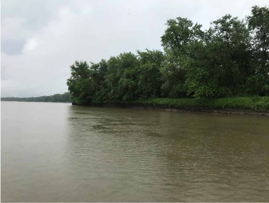
Figure 3: Looking upstream at upper end of Moore's Towhead right descending bank (39.893604°, -90.571933°).
