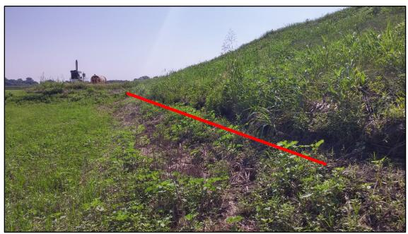
Figure 4. Typical Type III Erosion Damage (02-SEP-15).
