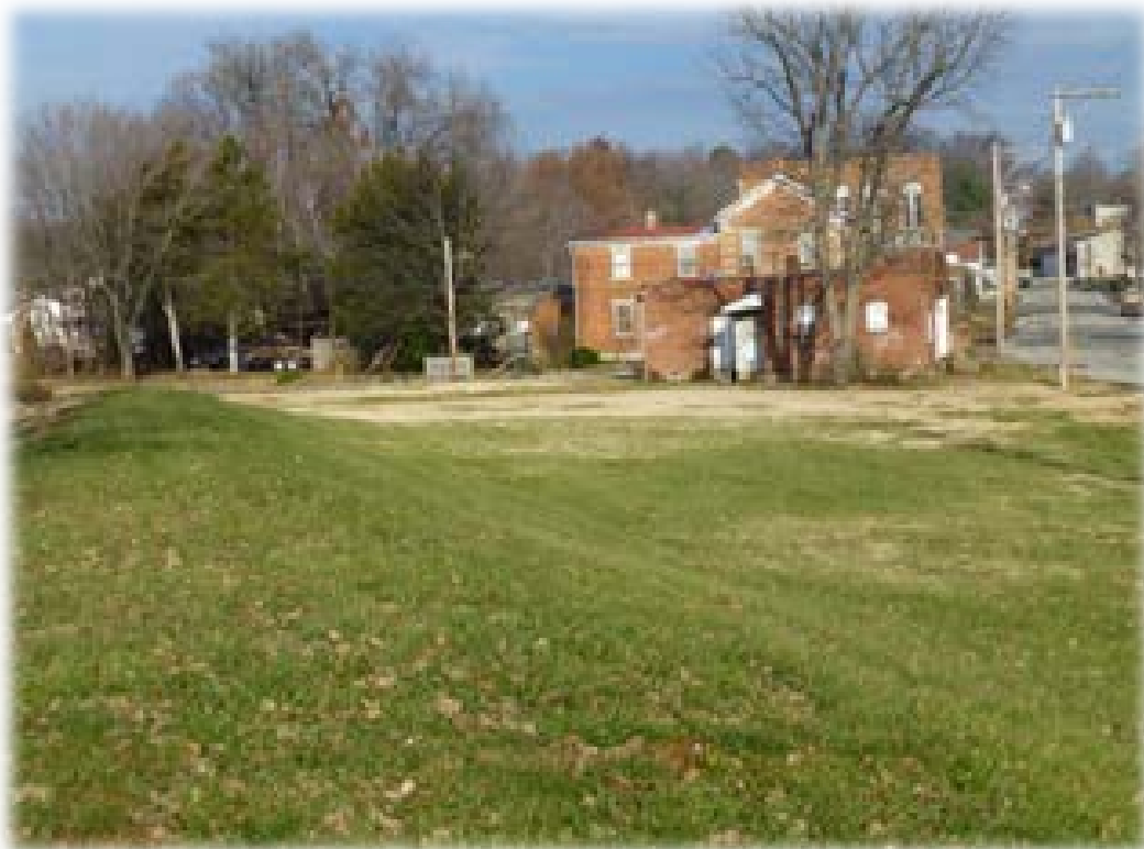
Figure 3-4. Existing Levee along the North Side of the North Gabouri Creek
