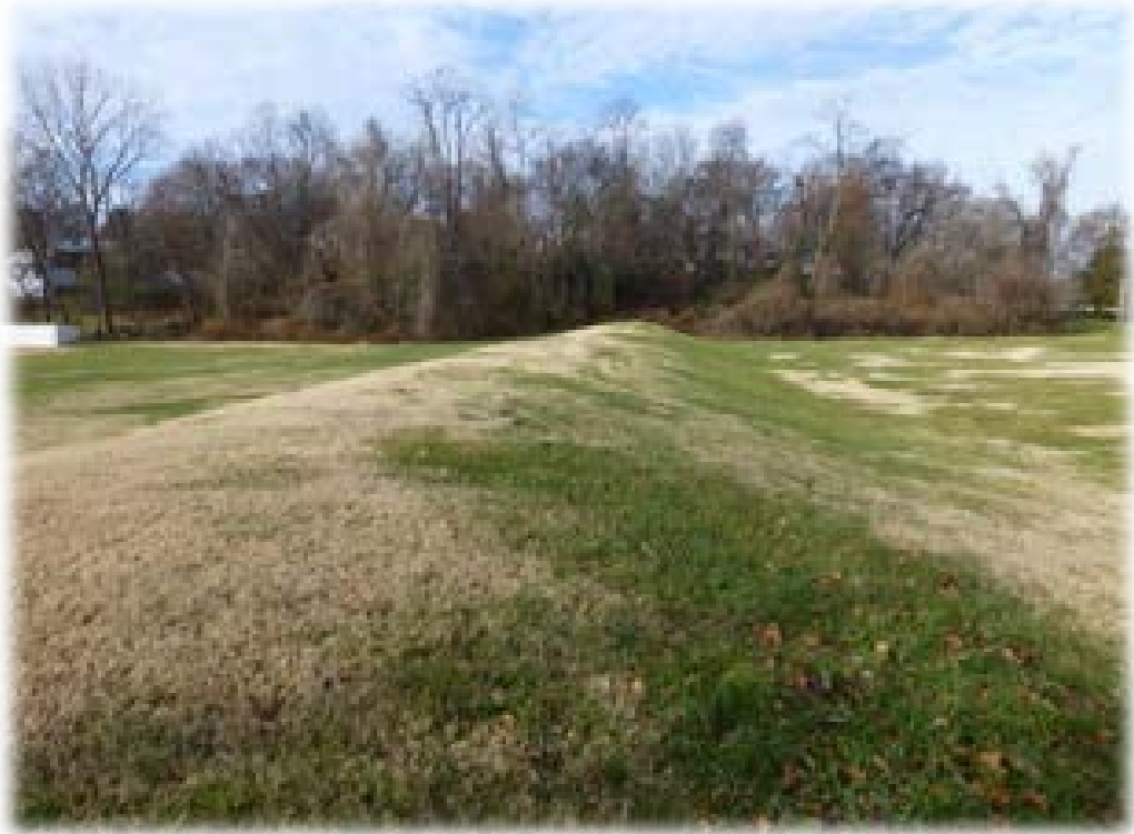
Figure 3-5. Existing Levee along the South Side of the North Gabouri Creek
