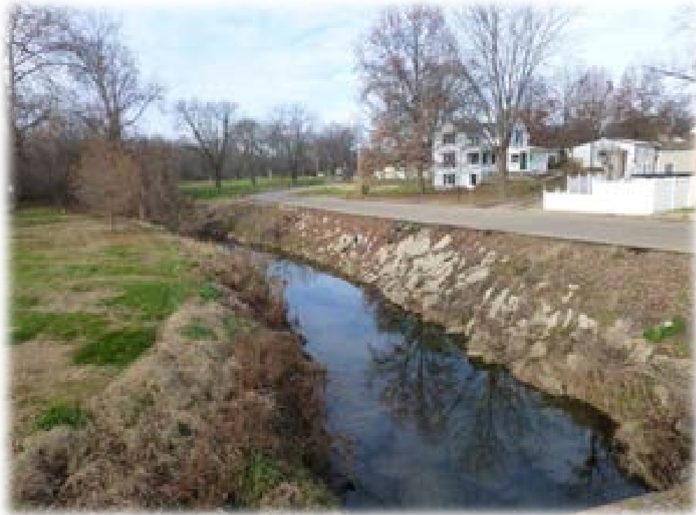
Figure 3-7. Creek bed along North Gabouri Creek around Sta. 50+00
