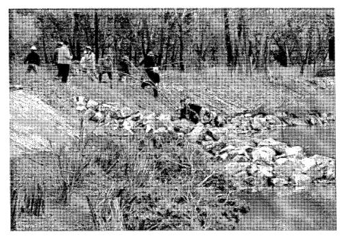
Figure 4. Incorporating irregular alignments, features such as spurs, and other habitat measures into a revetment can significantly improve habitat benefits
