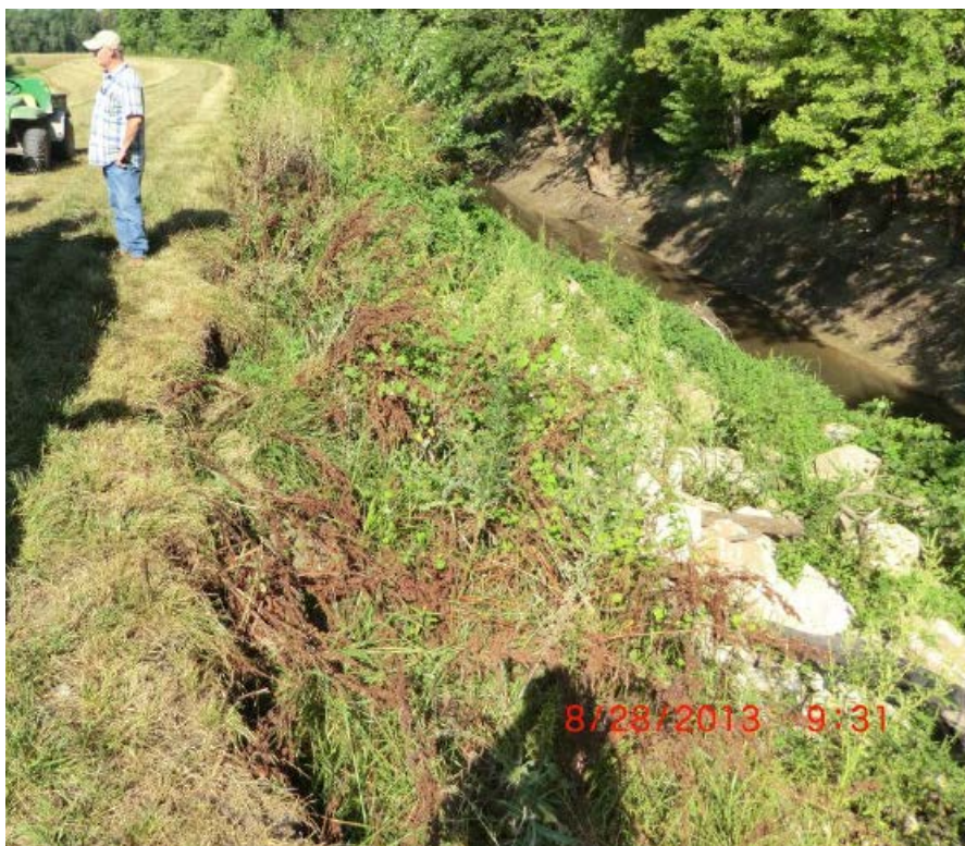
Figure 7 - Levee Scour and Slide Area along Cole Creek
