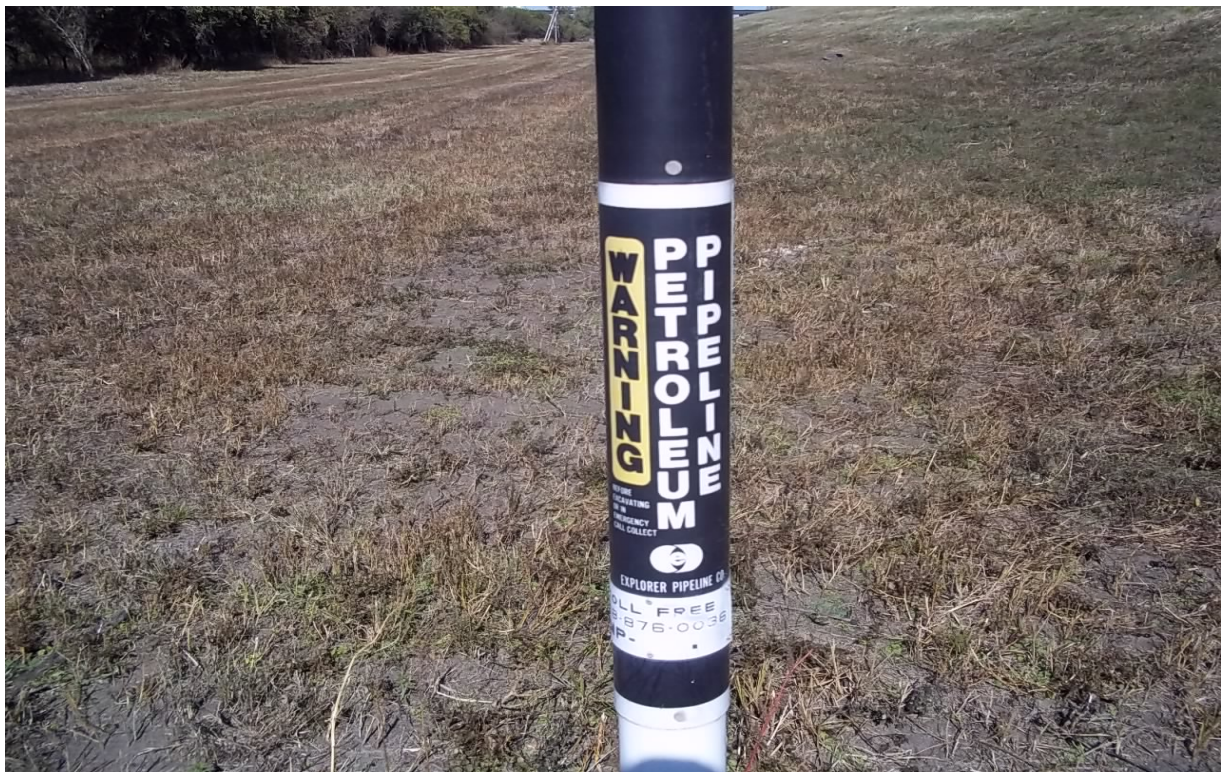
Photo 6. Petroleum pipeline on the west adjacent property to the subject site.
