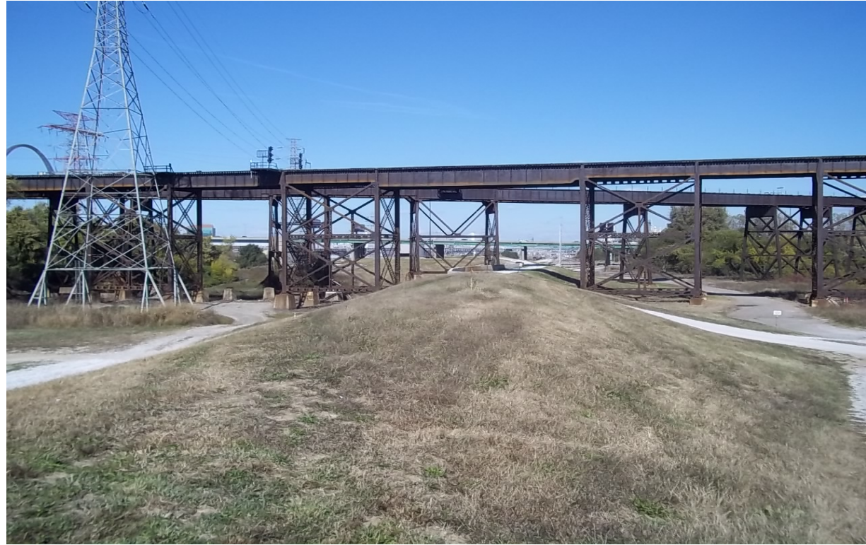
Photo 1. View to the north of the subject site.
