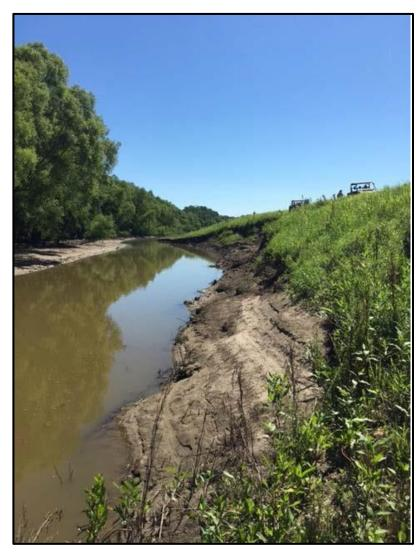
Figure 7. Photo of the levee slide at STA 728+20 to STA 732+40.
