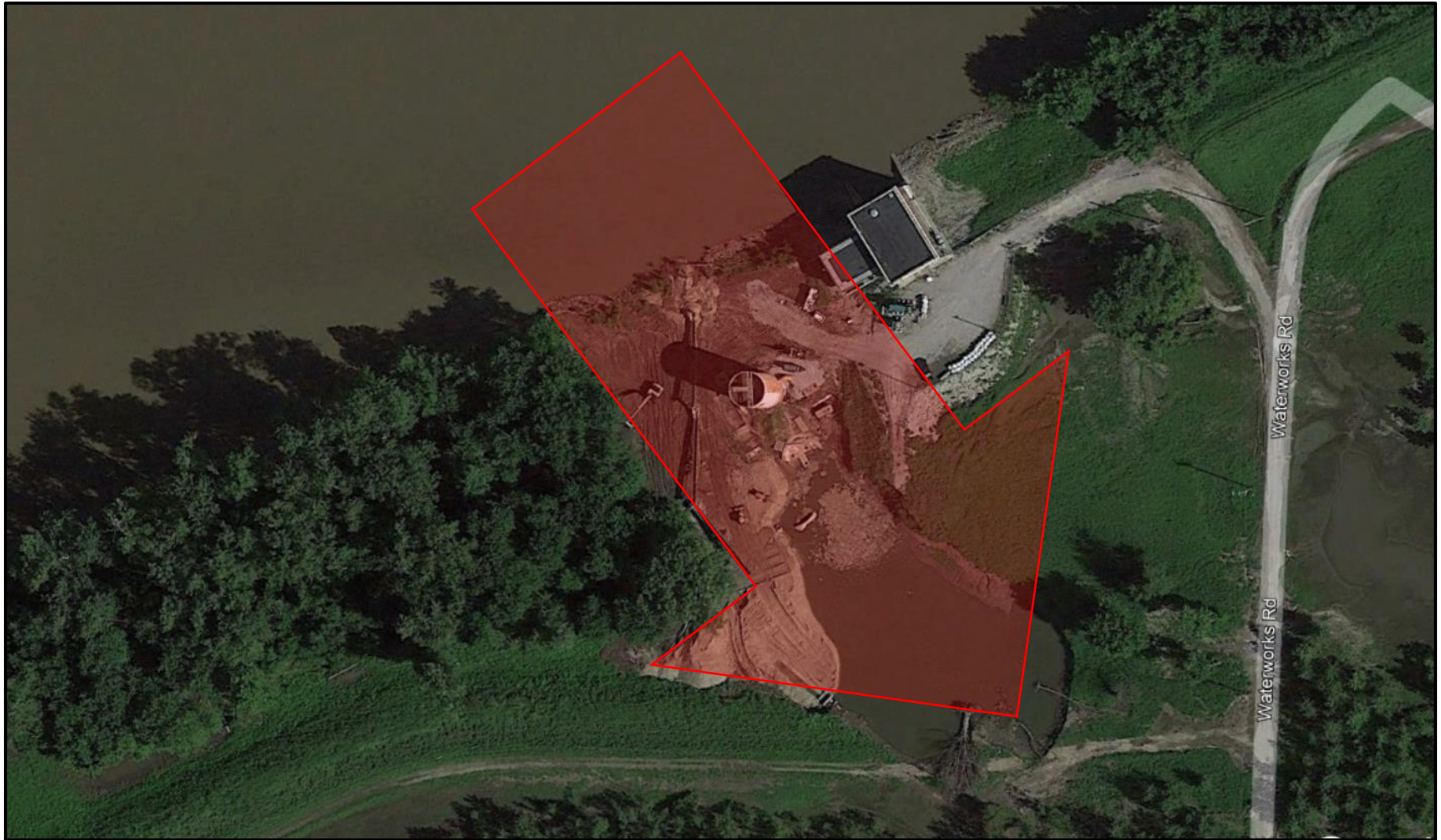
Figure 8. General location of levee breach due to 2019 flood.
