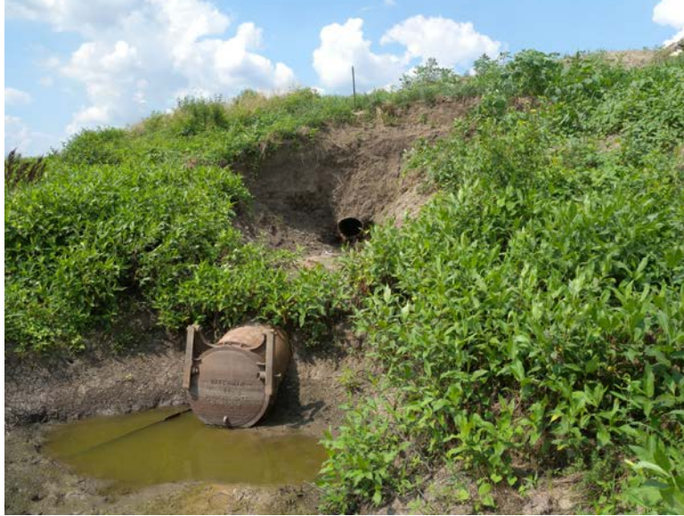
Figure 10 –Gravity Drain Failure (Area 3)
