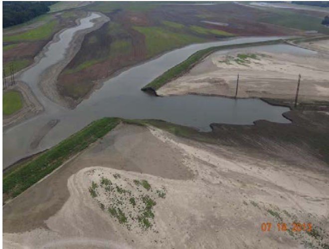
Figure 7 – Breach (Area 2)
