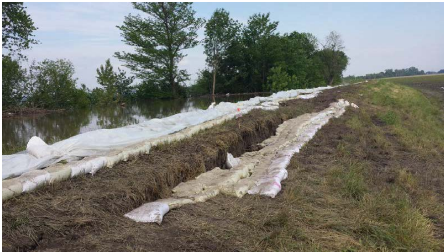
Figure 4 – Embankment Slide (Area 1)
