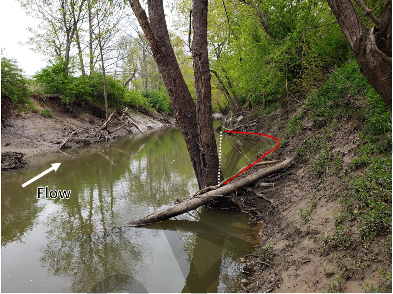
Figure 3. Streambank erosion adjacent to lagoons
