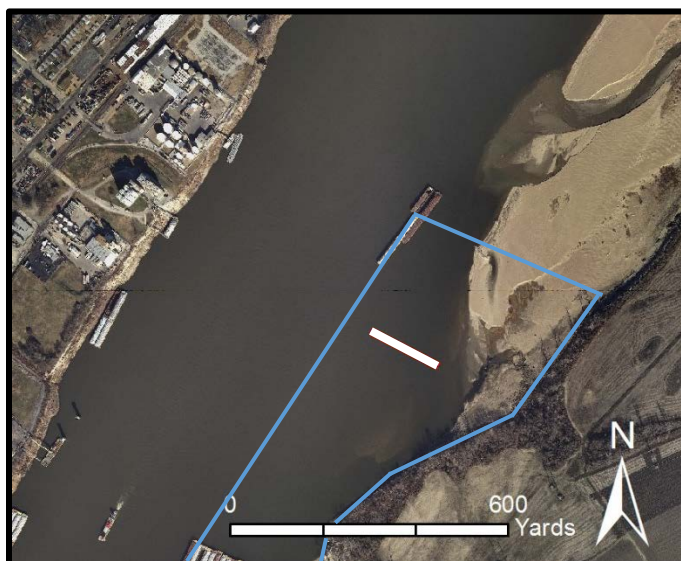
Figure 8. Aerial imagery of the Mosenthein Ivory-Landing Phase 4 work area, including the new rootless dike (white) and total area of influence (blue).
