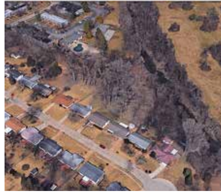
Palm Drive Properties and its cul-de-sac area require soil removal.
