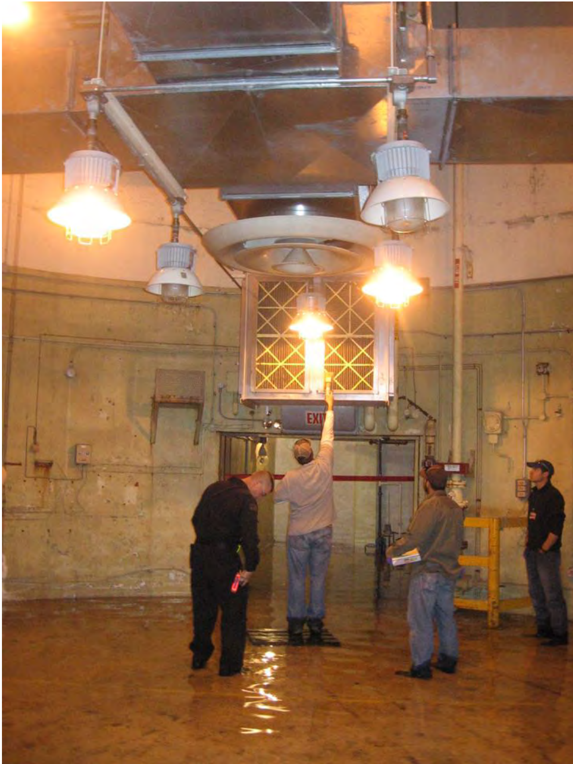
Figure 4-11. Photograph of the HVAC air filter in Building 1-63-6.
