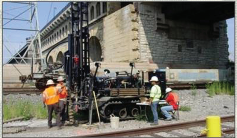
Above: Subsurface investigation at floodwall near Eads Bridge. Below: Heavy industry protected by the levee.
